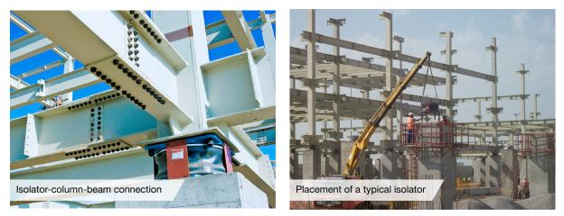
To determine the amount of movement it could withstand, Arup used real-time earthquake simulation modelling and LS-DYNA specialist software to test the building's integrity at 100<sup>th</sup> of second intervals. The results of 14 potential earthquake scenario tests showed that it could withstand an earthquake of magnitude 7.5-8.0, as measured on the Richter scale.
