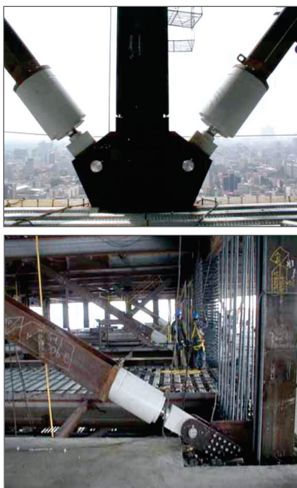
Fig.4: Damper installation
