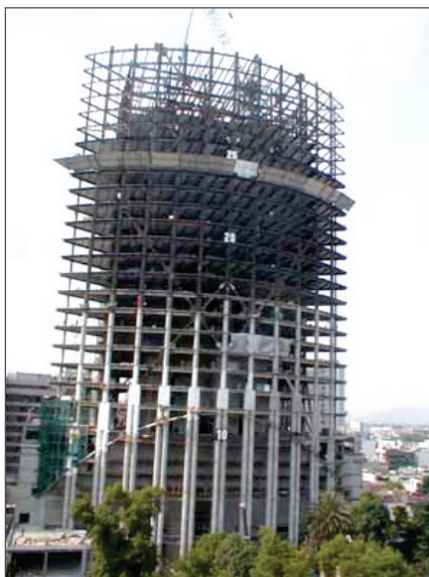
Fig. 3: Building frame during construction
