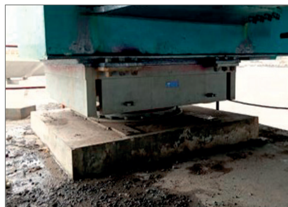
Fig. 14: Installed bearings
