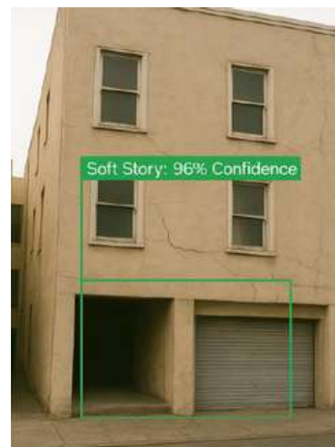
Figure 2 Model inference on a new image, successfully identifying and labeling a soft story vulnerability.
