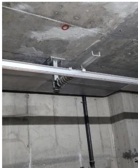
a) Finished post-installed connection
