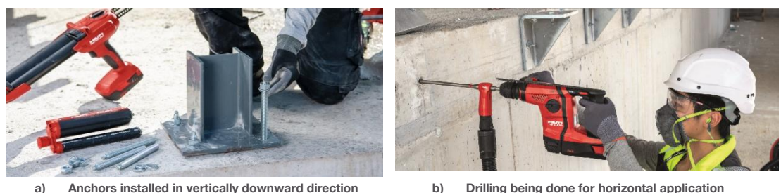
Fig. 8.12: Installation of adhesive anchors in different directions
