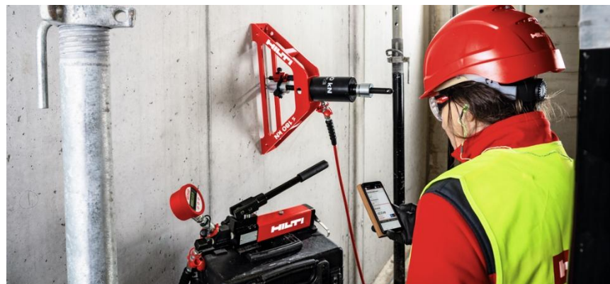
Fig. 8.18: Onsite testing by Hilti (unconfined tension setup)
