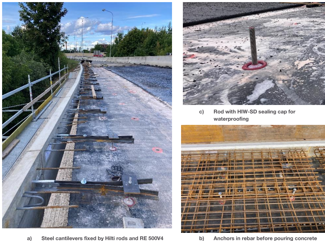
Fig. 9.10 Hilti Solution / products in bridge 231, Czech Republic
