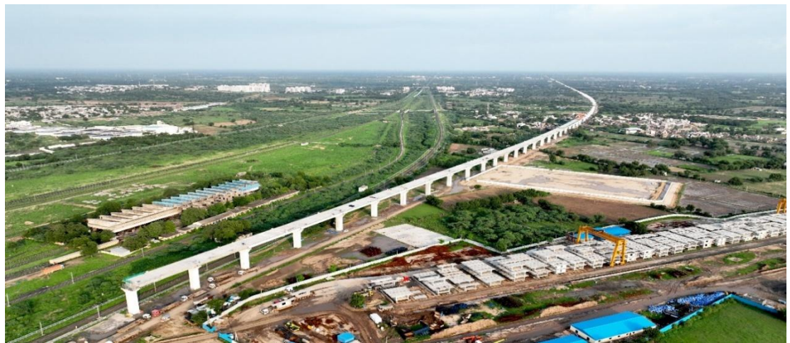
a) MAHSR viaduct portion
