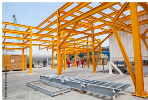
a) Primary steel column
