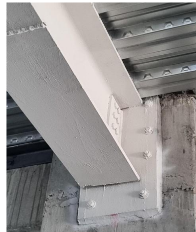
Fig. 6.10: Baseplate connection using group of anchors (4x2)
