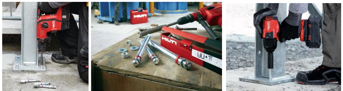
Fig. 8.9: Installation of mechanical anchors using setting tools and impact wrenches
