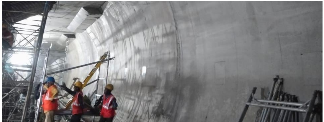
a) The structure at job site
