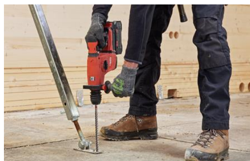
a) Drilling holes with a Rotary hammer
