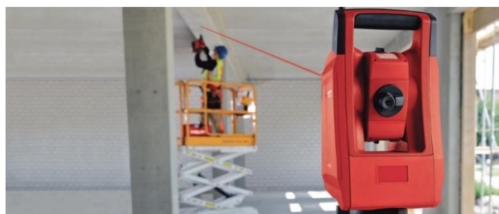
Fig. 8.4: Use of laser at a jobsite while positioning bore holes
