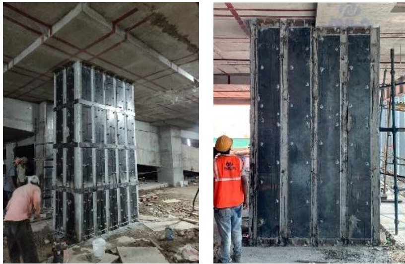
Fig. 8.3: Steel plate jacking of columns
