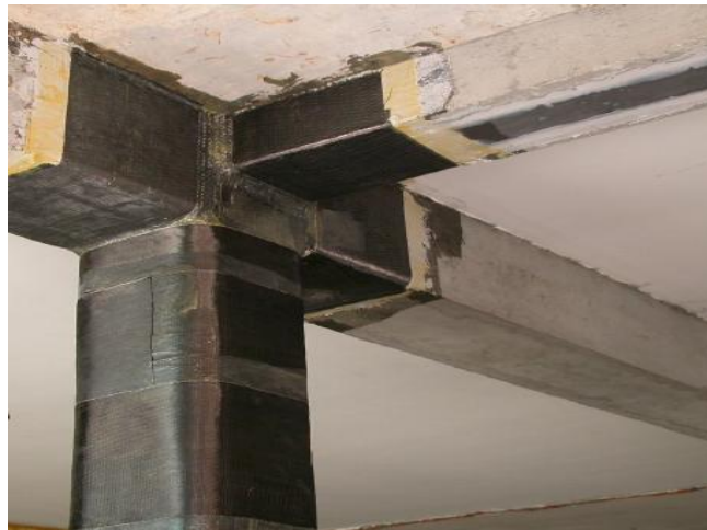
Fig. 8.5: FRP wrapping of beam-column joint
