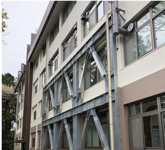
Fig. 8.7: Building strengthened with external braced frame
