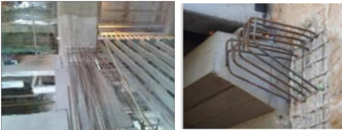
b) Column to slab/corbel
