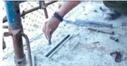
Step 8 – Sliding channel bolt into position
