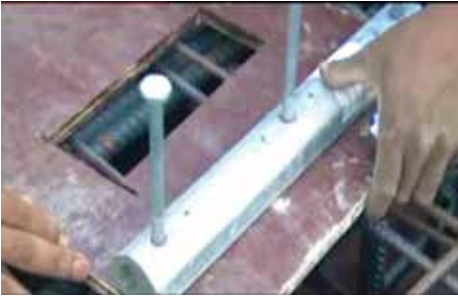
Step 3 – Nailing of cast-in anchor channel to wooden plank
