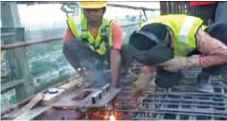
Step 5 – Welding of rebar support to existing reinforcement cage
