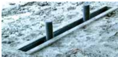
Step 9 – Securing fixture to the channel bolt
