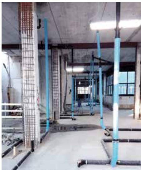
(b) Concrete jacking
