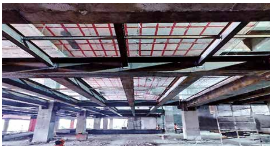
(b) Girder connections
