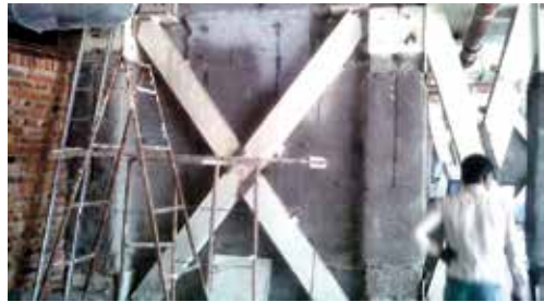
(b) Seismic bracing attachment
