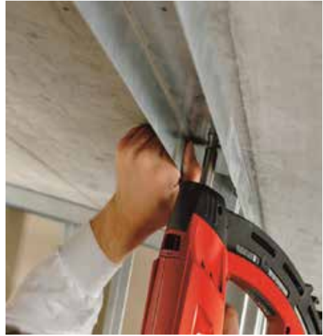
(f) Dry wall track fastening to concrete
