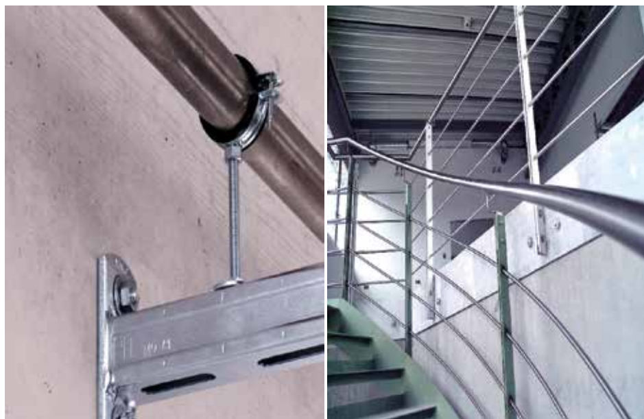
(a) Utility fixing
