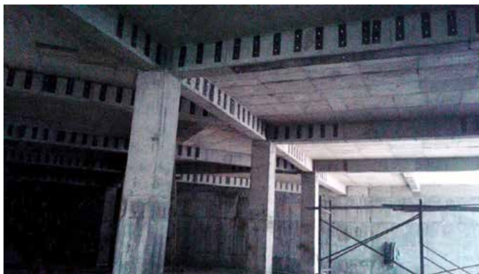
(c) Steel jacking for beam strengthening
