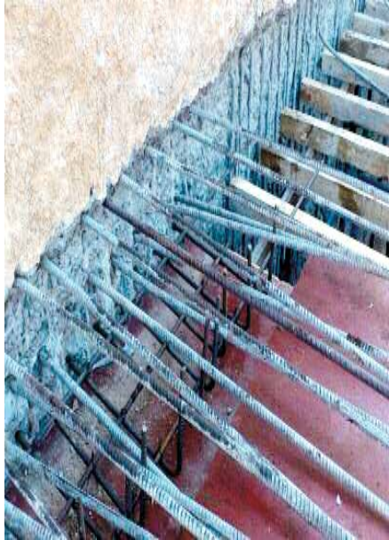
(b) Slab erection from D-Wall
