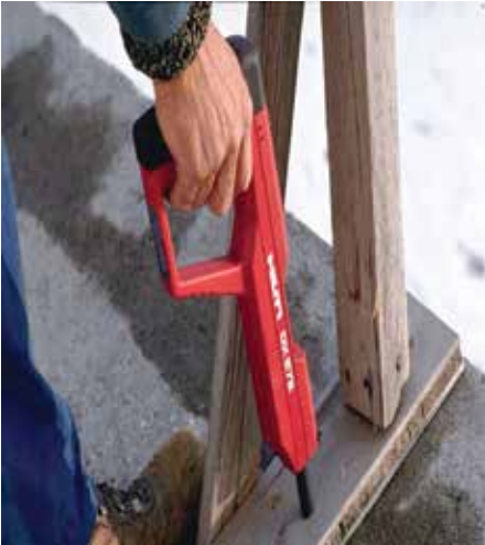
(e) Fastening of wooden batten to concrete
