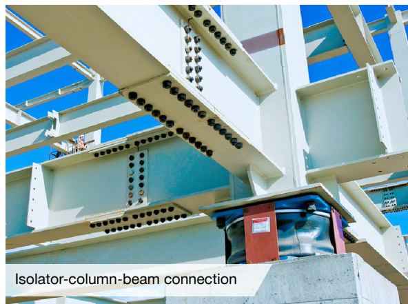
Placement of a typical isolator
