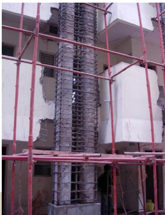
Fig. 4: Sharavati Hostel, IIT Madras (Courtesy: Hitech Concrete Solutions, Chennai)
