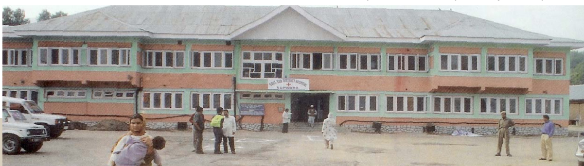
Fig. 3b: Civil Hospital at Kupwada, Kashmir (Courtesy: Building Materials and Technology Promotion Council, New Delhi)
