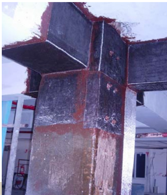
Fig. 6: FRP wrapping with near surface mounted plates at Apollo Proton Therapy and Cancer Hospital, Chennai (Courtesy: Sanrachana Structural Strengthening Pvt. Ltd., Larsen & Toubro Construction)
