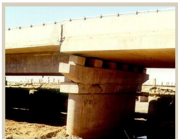
Fig. 3: Bridge between Surajbari and Bhachau
