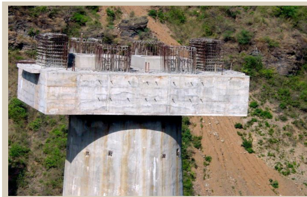
Fig. 21: Details at restrained bearing over abutment
