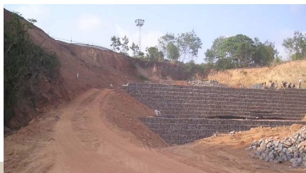
Fig. 5: Strengthening of unstable slopes using gabions at Mangalore Refinery
