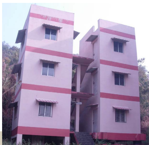
Fig. 7: Base isolation units placed in the right wing of a prototype building (Courtesy: Sajal K. Deb, Indian Institute of Technology Guwahati)
