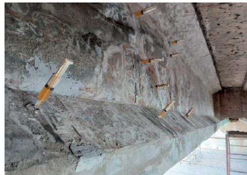
Fig. 8: Crack Repair by Epoxy Injection
