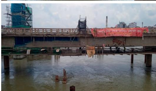
Fig. 7: Suspended Staging for Under-Bridge Repairs
