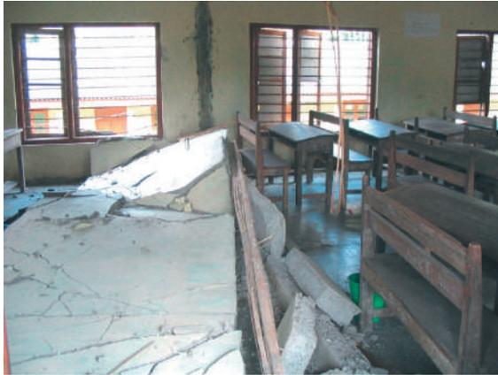
Fig. 11: Slender masonry walls dislodged due to out-of-plane instability
