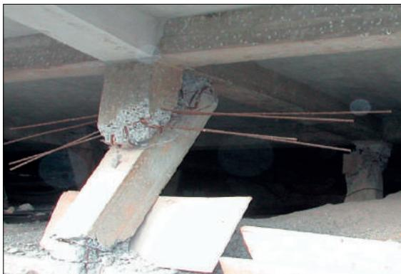
Fig. 9 Three storied RC framed building collapsed
