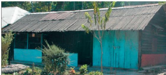
Fig. 8: Single-story wood house in Port Blair with light roof had no damage
