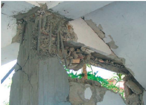
Fig. 12: Building showing severe cracking and damage to soft ground storey
