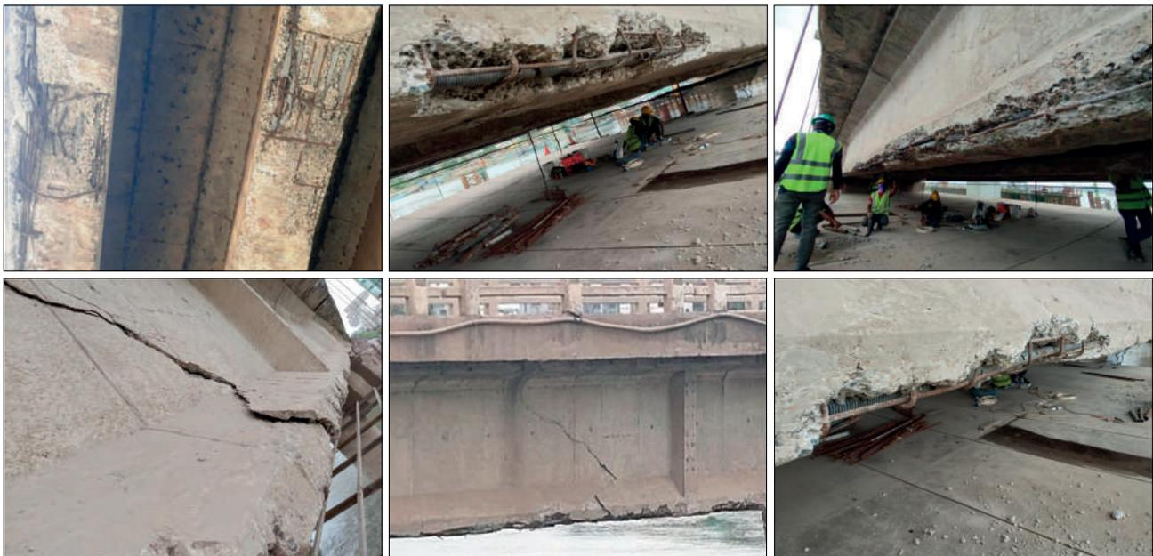
Fig. 5: Extent of damage from the field observation
