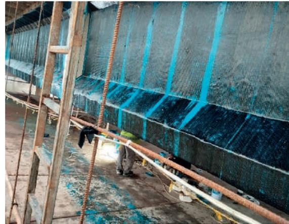
Fig. 12: Strengthening of the girder by installing CFRP fiber wrapping.
