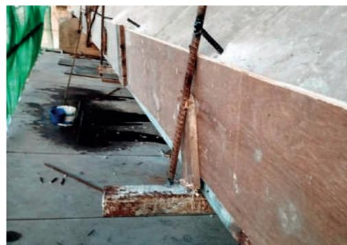
Fig. 9: Spalling repair using Micro-Concrete
