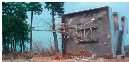
Fig. 16: Laterally toppled three-story seaport traffic control tower at Hut Bay
