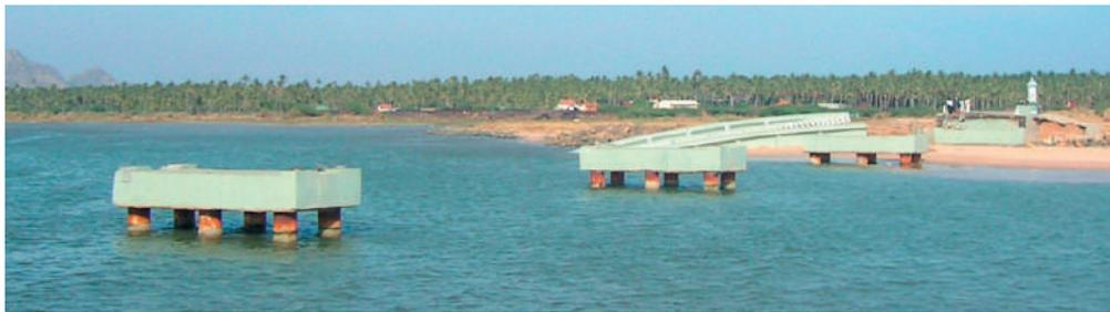
Fig. 14: Loss of spans of the four span RC bridge at Melmannakudi in Tamil Nadu
