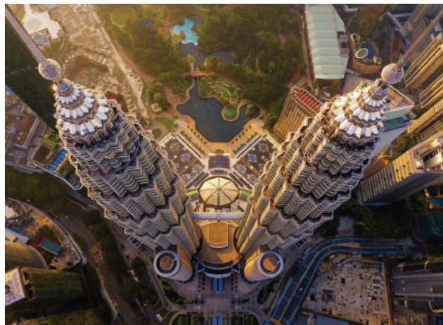
The towers were built on a soft soil foundation, which posed a significant engineering challenge. The foundation system consisted of a 4.5-meter-thick piled raft supported on rectangular friction piles, varying in depth from 40 meters to 105 meters and each foundation consisted of 104 barrettes.
